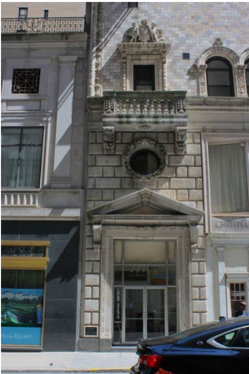
Figure 5. Façade (west elevation): Left (north) entrance.
