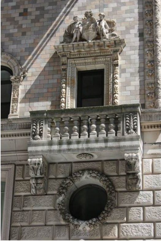
Figure 6. Façade (west elevation): Detail of ornament over left (north) entrance, 2nd and 3rd floors.
