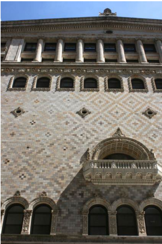
Figure 7. Façade (west elevation): 3rd through 8th floors.
