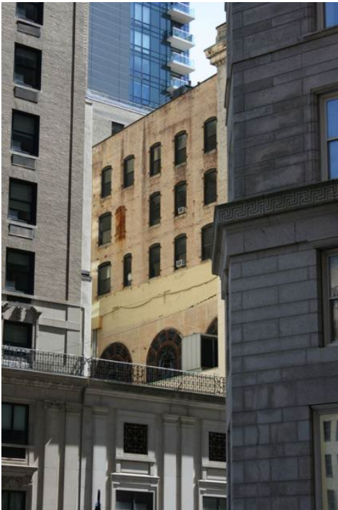
Figure 9. North elevation (light-ochre color wall in center of image), upper floors.
